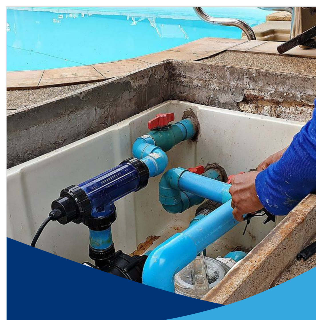
AUTOMATIC SWITCH REPLACEMENT (PUMP ROOM)
