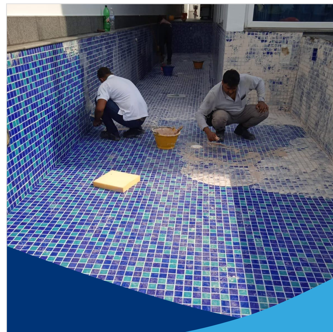
EPOXY GROUTING SERVICE
